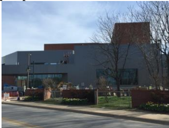
Above: From West Avenue looking at the new West Avenue Lobby windows (left) and Starr Theater window (right)
